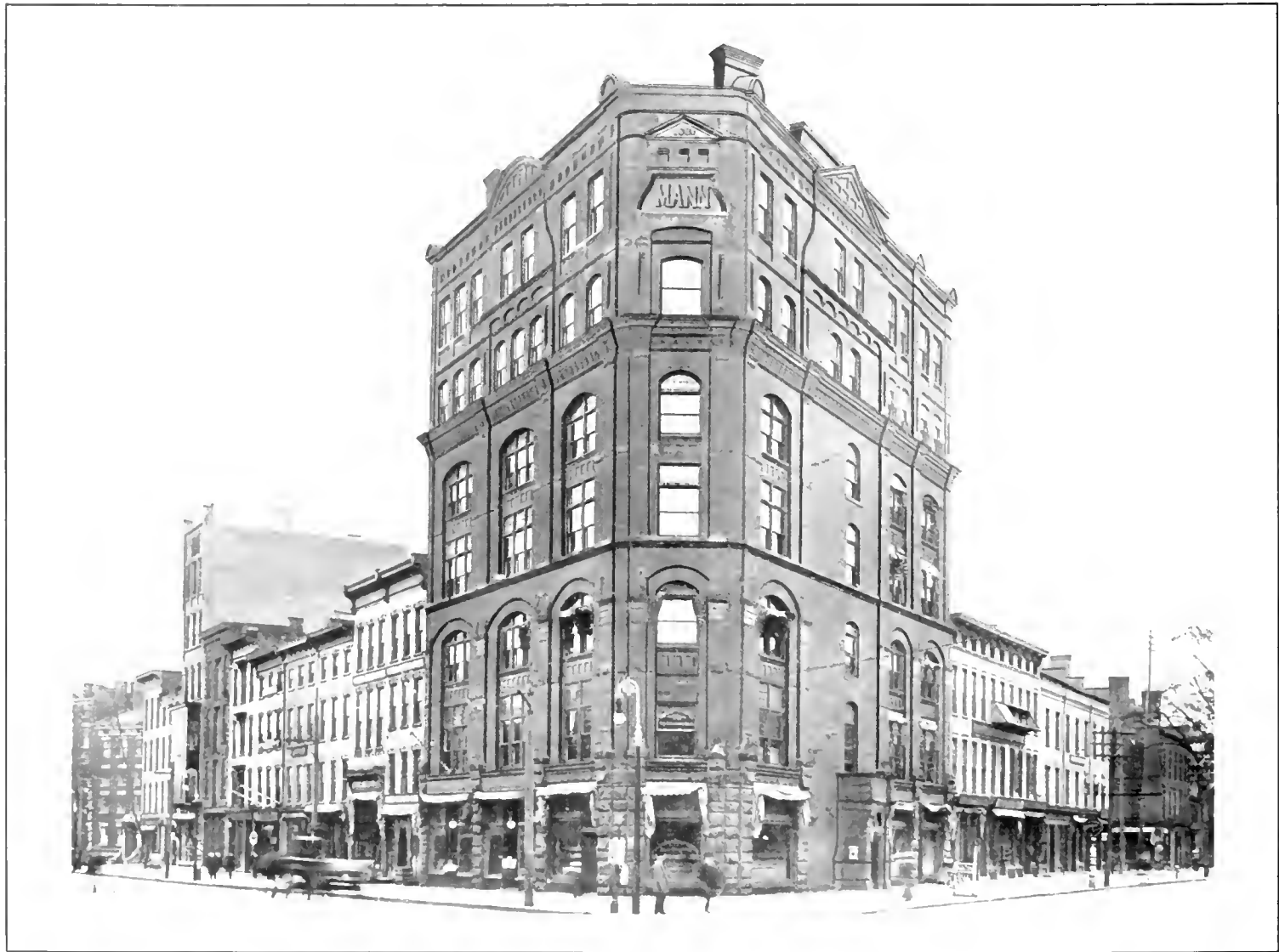
MANN BUILDING—GENESEE STREET, CORNER OF BROAD
